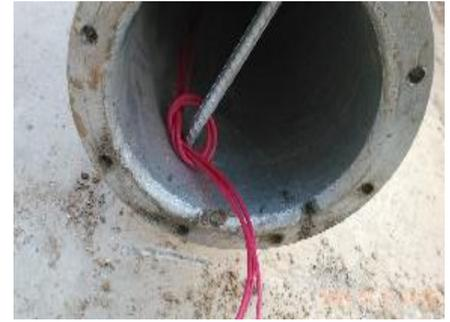
2). Keep the base on bottom of tower flat, put washer on the screw of anchor, tight the nut. Put cable through the tower; connect the two sections of tower and the base. Lay on pit A.
